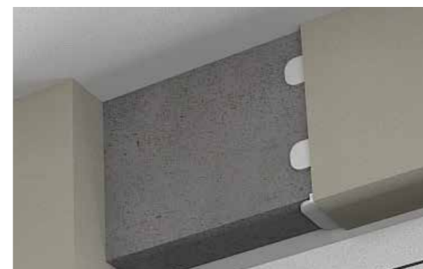
DRY-PLASTERED LINTEL CLADDING
