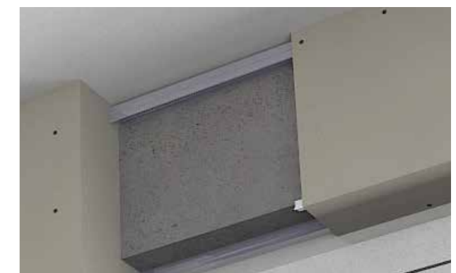
LINTEL CLADDING WITH SUBSTRUCTURE
