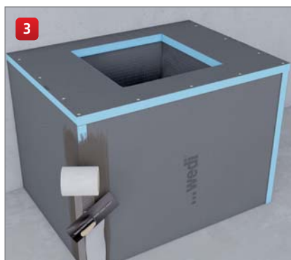
... reinforce butt joints ...
