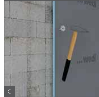
C Place wedi Tools metal dowels in the holes and hammer in after the mortar has fully dried.
